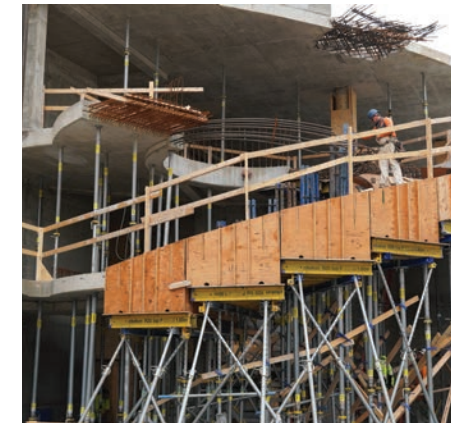
JUNE 2024 Form work for the spiral staircase in the new front of house expansion begins.
