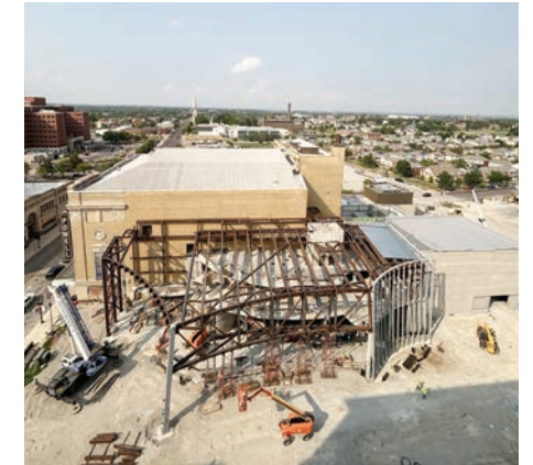
JULY 2024 Crews begin building the steel shell that will envelop the expansion.
