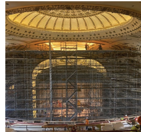
MARCH 2024 Scaffolding fills much of the auditorium as cleaning and painting begins.
