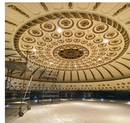
AUGUST 2024 Powell Hall’s iconic dome is cleaned and repainted.
