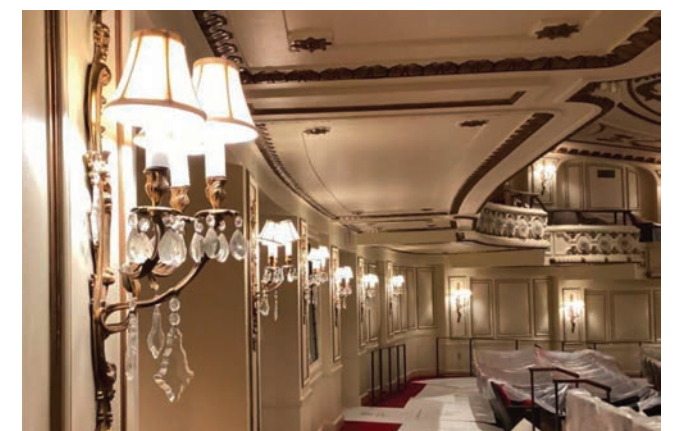
JULY 2025 Light fixtures are reinstalled in the auditorium.
