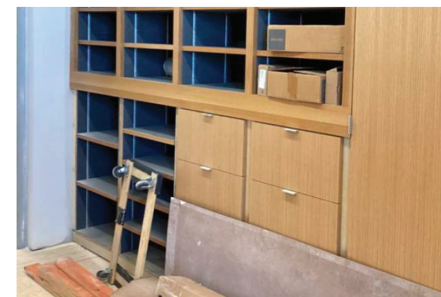
APRIL 2025 Instrument storage is installed.
