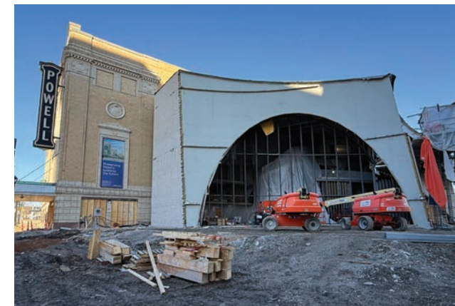
FEBRUARY 2025 The new main entrance is installed.
