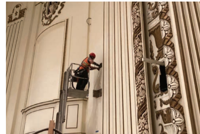
OCTOBER 2024 Crews updated the electrical work around the proscenium in the auditorium.
