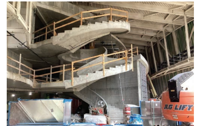
OCTOBER 2024 The spiral staircase takes shape in the new Berges Family Foundation Grand Lobby.
