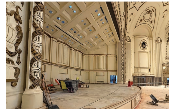
MARCH 2025 The stage flooring is removed to make way for the new white oak floor.
